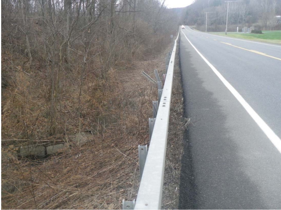
Photo 5: East Bridge Rail (looking south)
