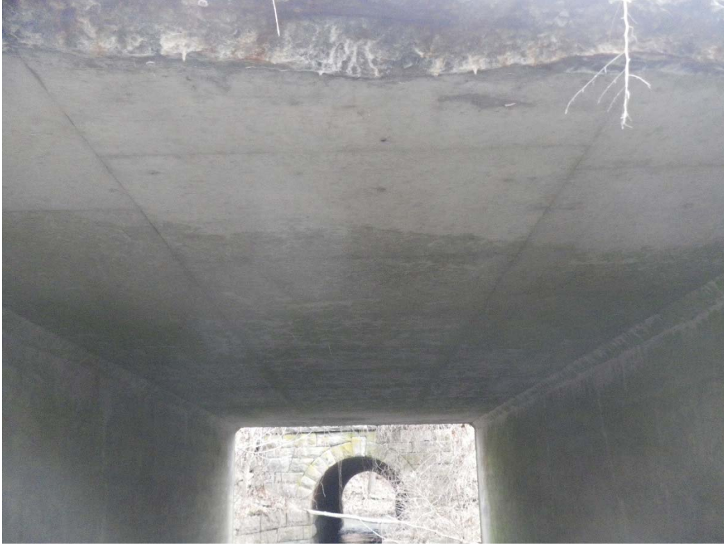
Photo 21: Top Slab (looking east)
