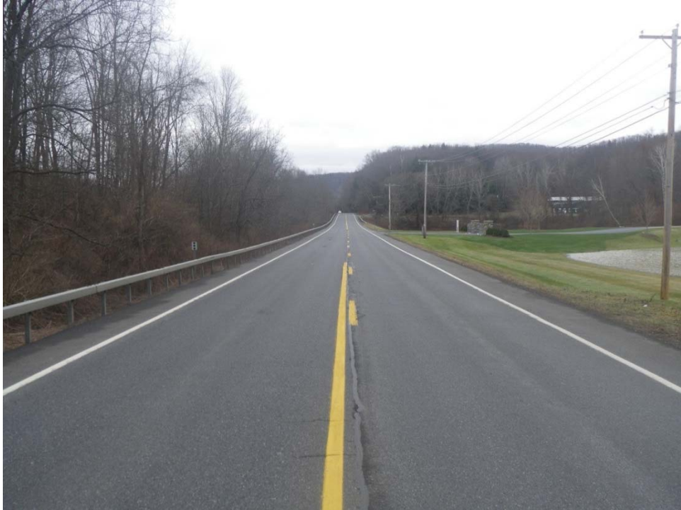
Photo 2: Route 22 (looking south)
