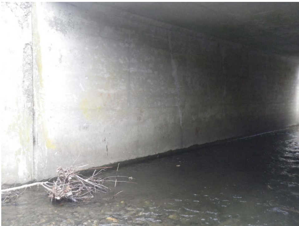
Photo 16: North Leg (looking east)
