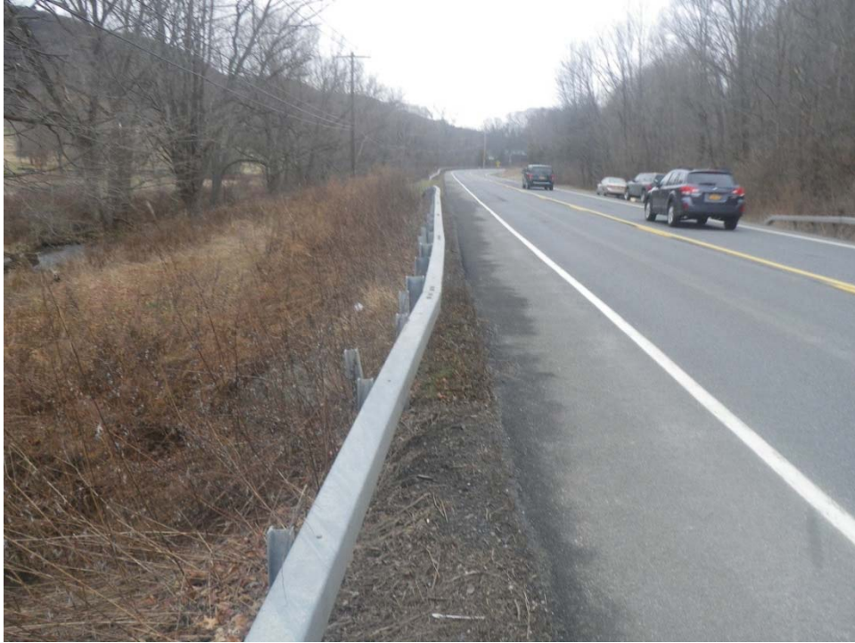
Photo 7: West Bridge Rail (looking north)
