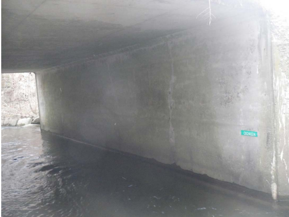
Photo 18: South Leg (looking east)
