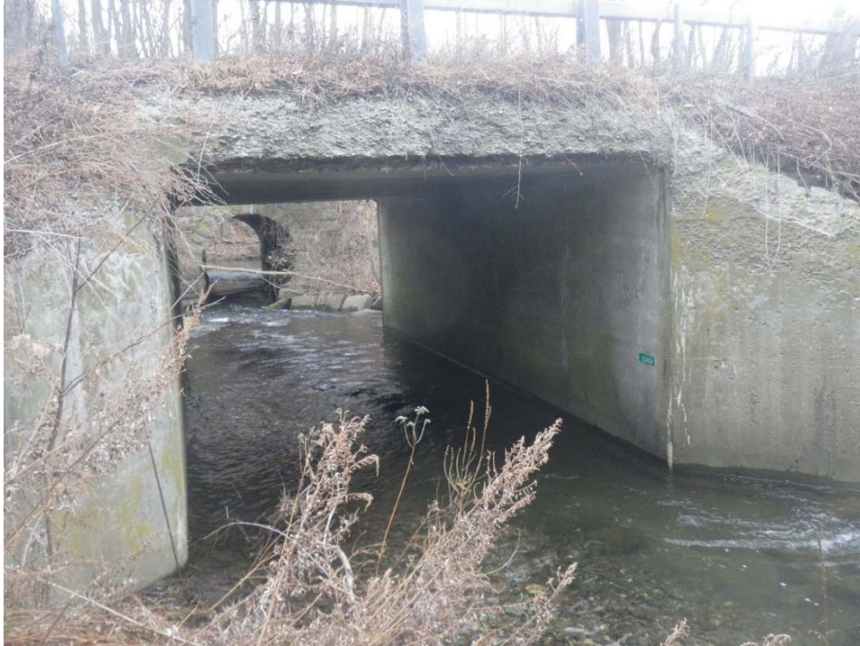
Photo 8: Box Culvert – West Fascia
