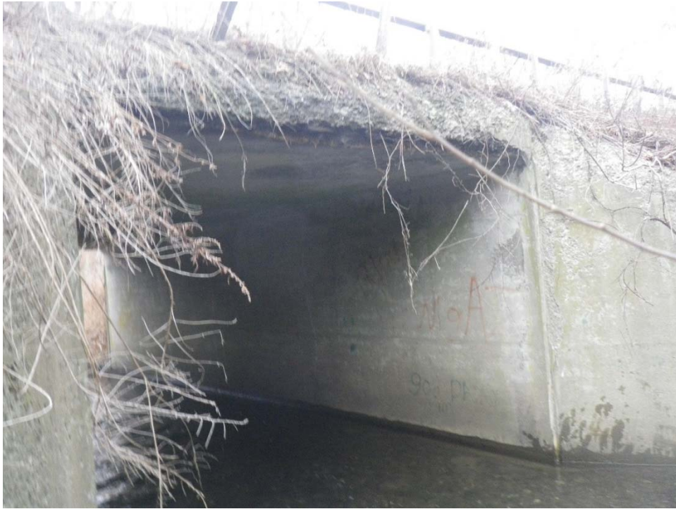
Photo 11: Box Culvert – East Fascia
