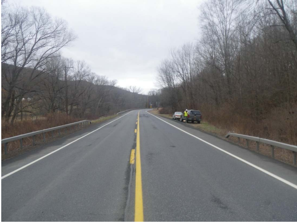
Photo 1: Route 22 (looking north)
