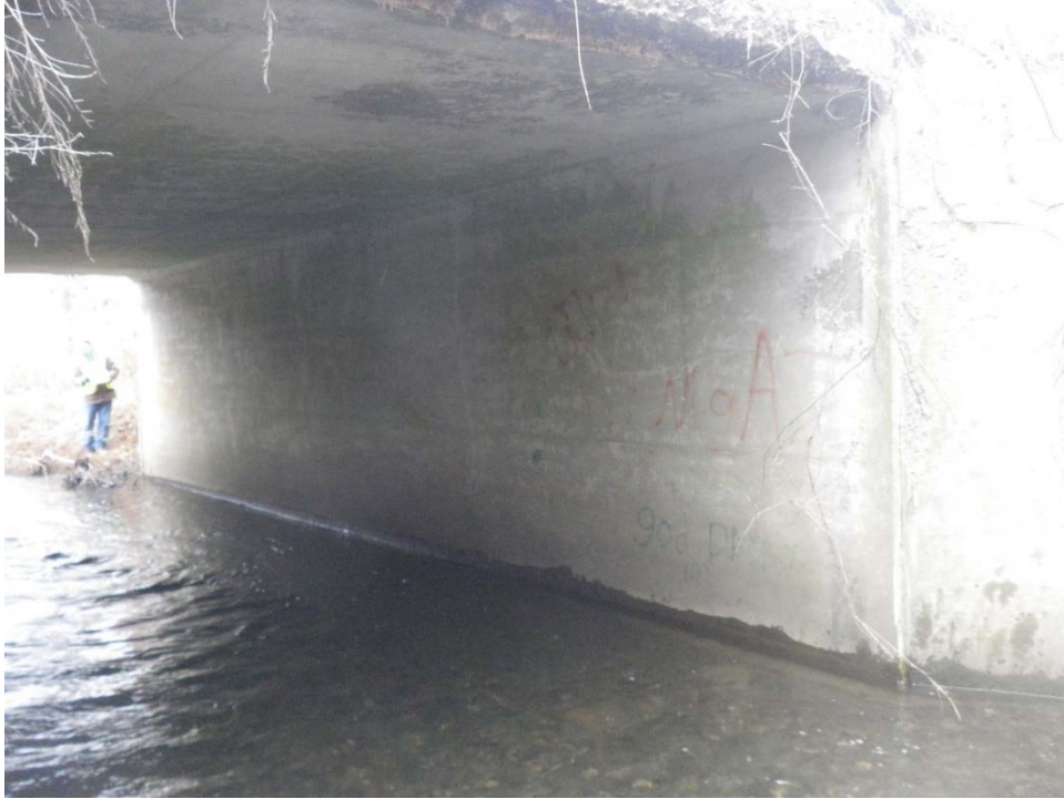
Photo 17: North Leg (looking west)
