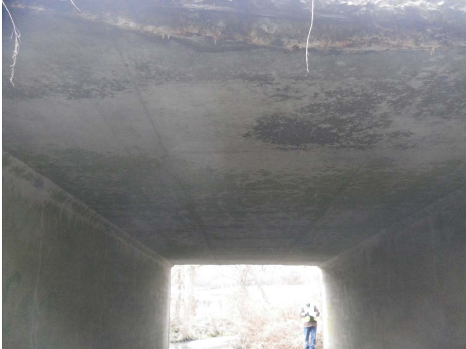
Photo 20: Top Slab (looking west)
